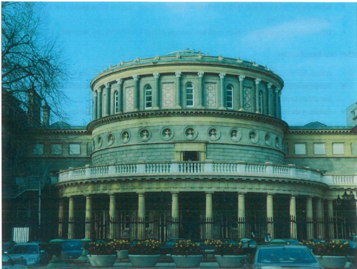
Figure 14. National Library of Ireland Fronting the Oireachtas Car Park
