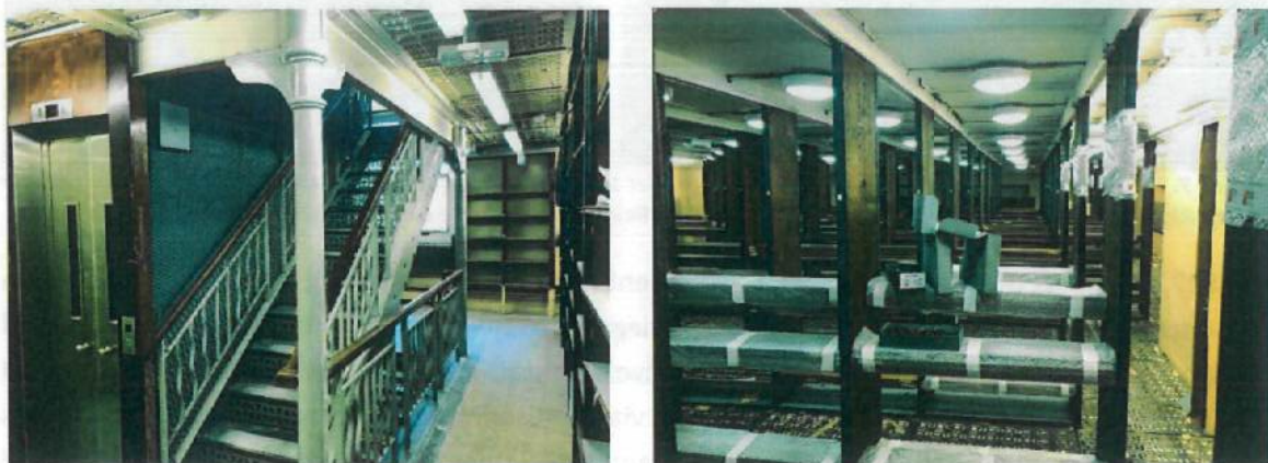
Figure 5. Cast iron staircase in west wing and structural shelving with cast iron floor deck Images: NIAH Record
