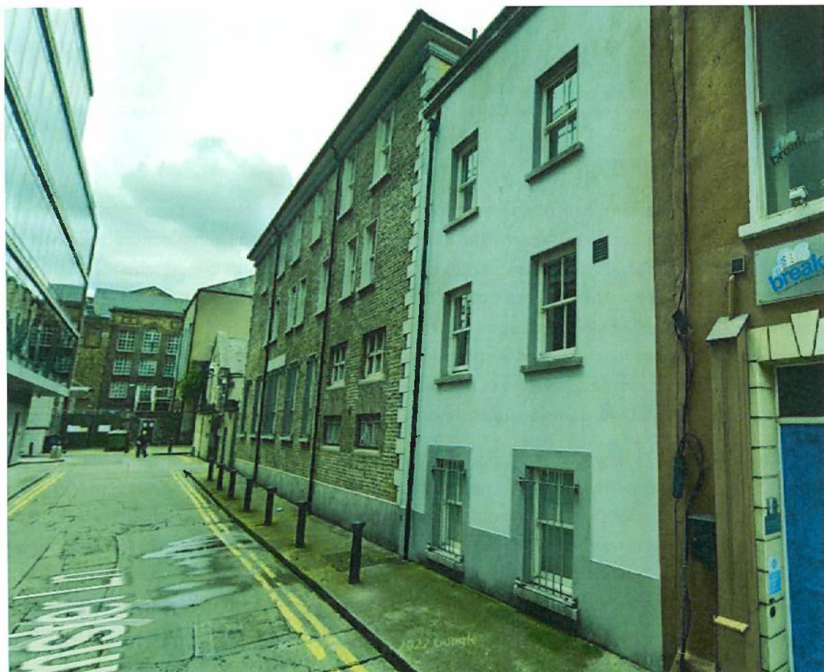
Figure 10. Racquet Hall (Brick) with Extension (Grey), Leinster Lane
